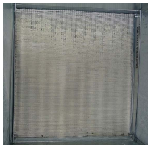
FIGURE 1 - EXAMPLE HEAT EXCHANGER AT FAILURE
